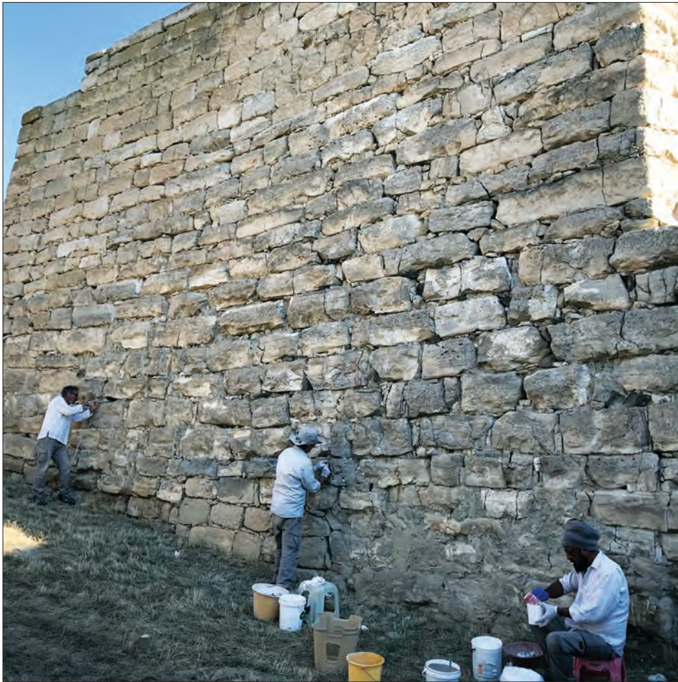
Figure 6: The Early Phrygian citadel's East Gate (9th century BCE): conserving the south wall of the North Court, looking northwest. Photo by Brian Rose.
