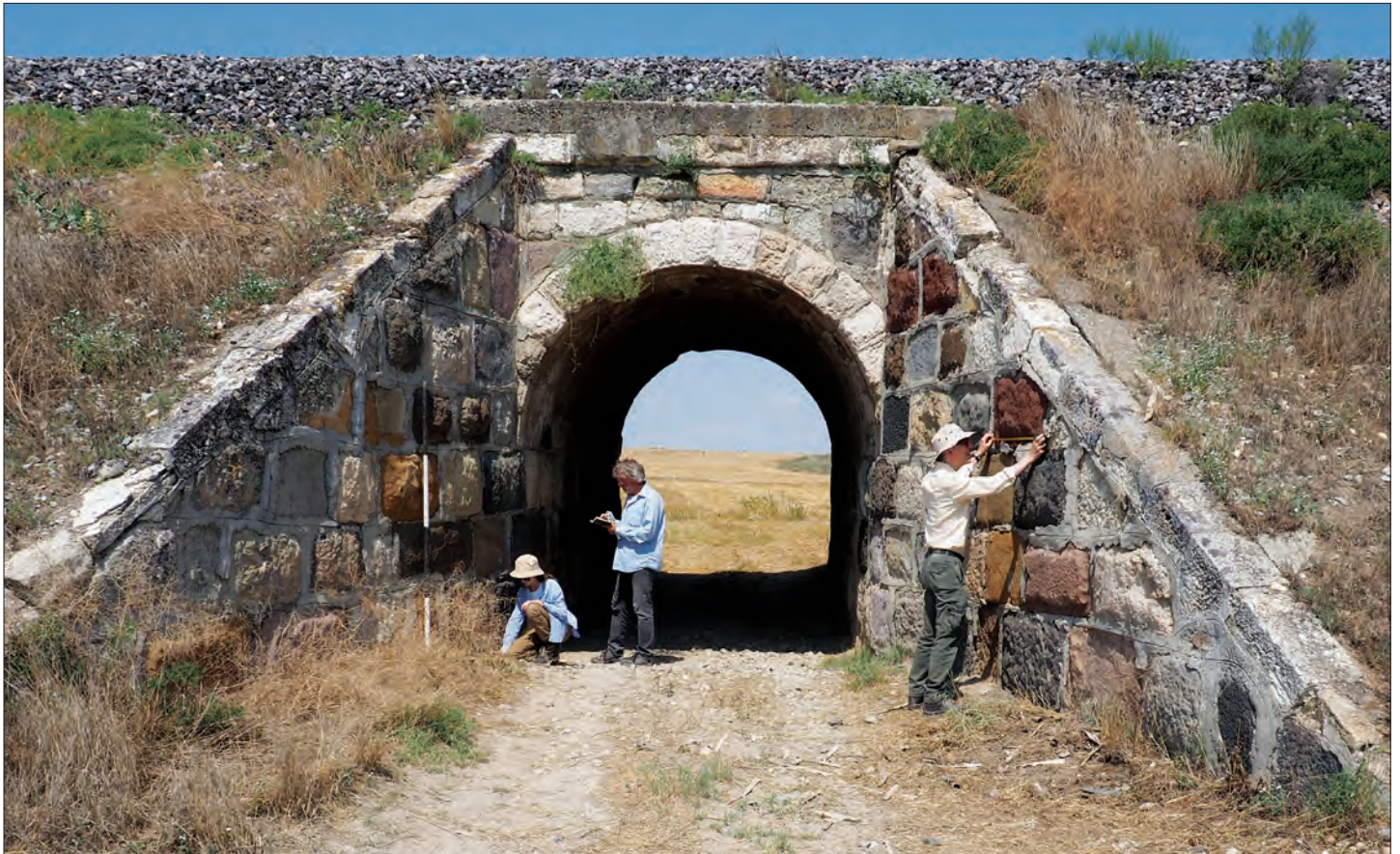
Figure 33: Late 19th century railroad bridge near Gordion with reused polychromatic Middle Phrygian (8th century BCE) stones, perhaps from the citadel's South Gate. Photo by Gebhard Bieg.
