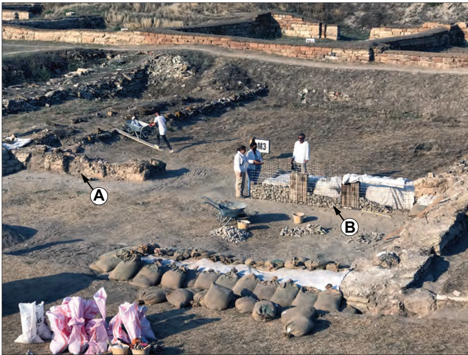
Figure 9: The conservation of Megaron 3 (9th century BCE), looking southwest. The ruined state of the megaron's dividing wall is visible at left (A). The wire, stone, and wood reconstruction of the wall is visible at right (B). The Terrace Building can be seen at the top. Photo by Brian Rose.
