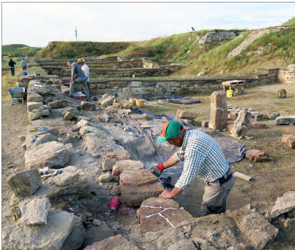
Figure 7: Conservation of the damaged walls of unit 7 of the Terrace Building (TB-7), looking southeast. The new security camera is the tall, slender looking object visible on the skyline at left. Photo by Elisa Del Bono.
