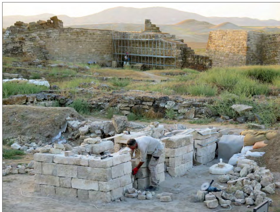
Figure 6: The new stone encasement around the damaged walls of Megaron 3, with the citadel's East Gate at top, looking southeast. Photo by Elisa Del Bono.
