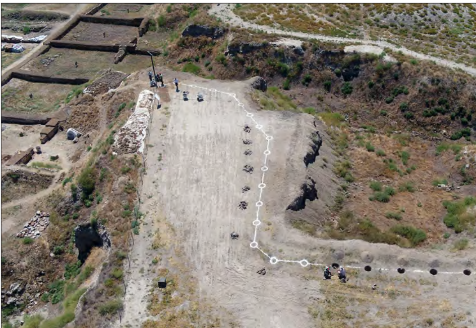
Figure 9: Installation of the new fence on the Visitor Circuit, looking south. The Terrace Building is at upper left. Photo by Ali Can Kırcaali and Zekeriya Utğu.
