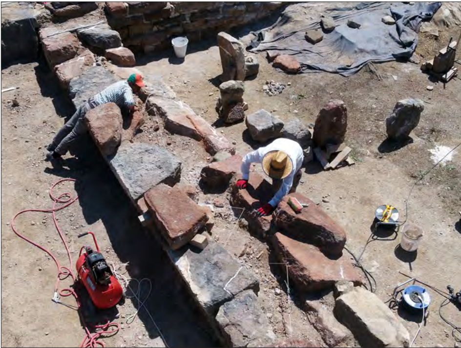
Figure 8: Conservation of the damaged walls of unit 7 of the Terrace Building (TB-7), looking southeast: insertion of steel cables through the core of the wall to secure the facing stones. Photo by Elisa Del Bono.
