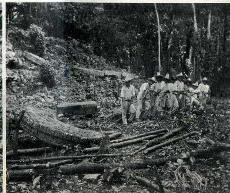
Below: Moving the top of Altar 1. Sixteen of the massive stone monuments, including stelae, were removed by comparatively primitive methods; they were then boxed, sometimes in sections, hauled by ox team over a road made for the purpose, thirty-five miles to the river below impassable rapids; from there they were floated by raft through a smaller rapid to the nearest port, and thence by steamers to Philadelphia
