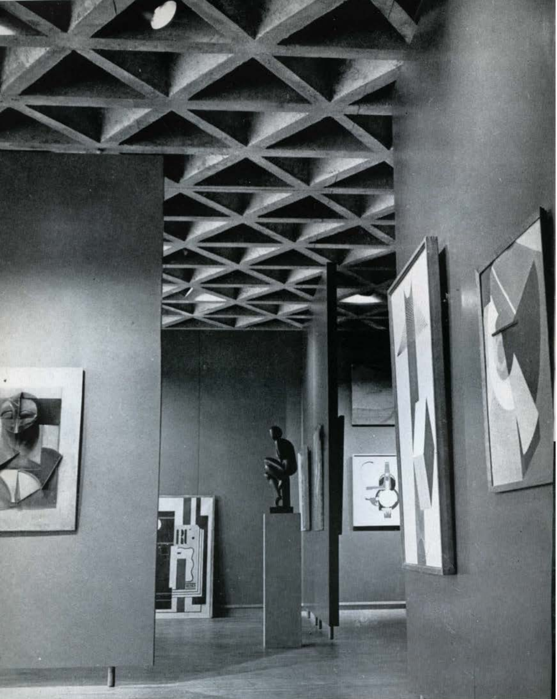
One of the rare examples of modern design for museum buildings is Yale's new Art Gallery and Design Center. Movable "pogo-panels" conceived by George Howe make a very flexible exhibit area. Details of design provided for sound-proofing, air conditioning, and flexible lighting equipment.
