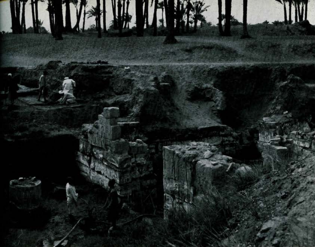
Fig. 2. The façade of the Sanctuary and the dig to the south of the colonnade ("A" in general map), in the middle of March, 1955, seen from N.E. The pump being operated in front of the entrance to the Sanctuary was not successful in draining the lower level.
