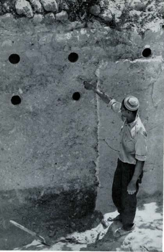
Fig. 22. Plaster removed from large reservoir used in Roman and Arab times, showing Roman jars imbedded in the masonry of the wall.
