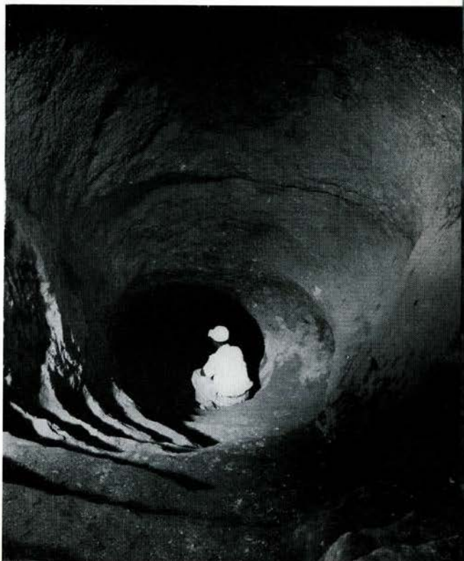
Fig. 6. First section of the tunnel bored through solid rock, looking down to the round opening which leads to the reservoir.
