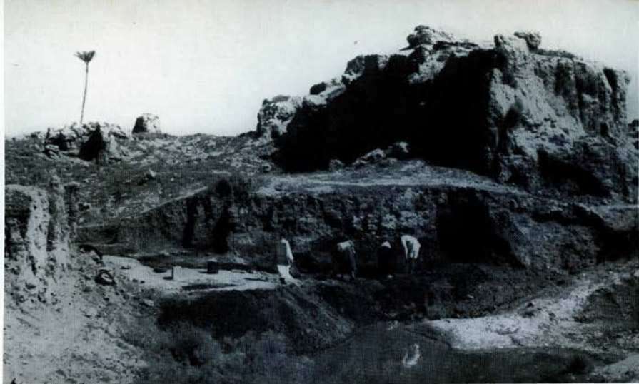
Fig. 6. Trial digging at Merenptah's South Portal.
