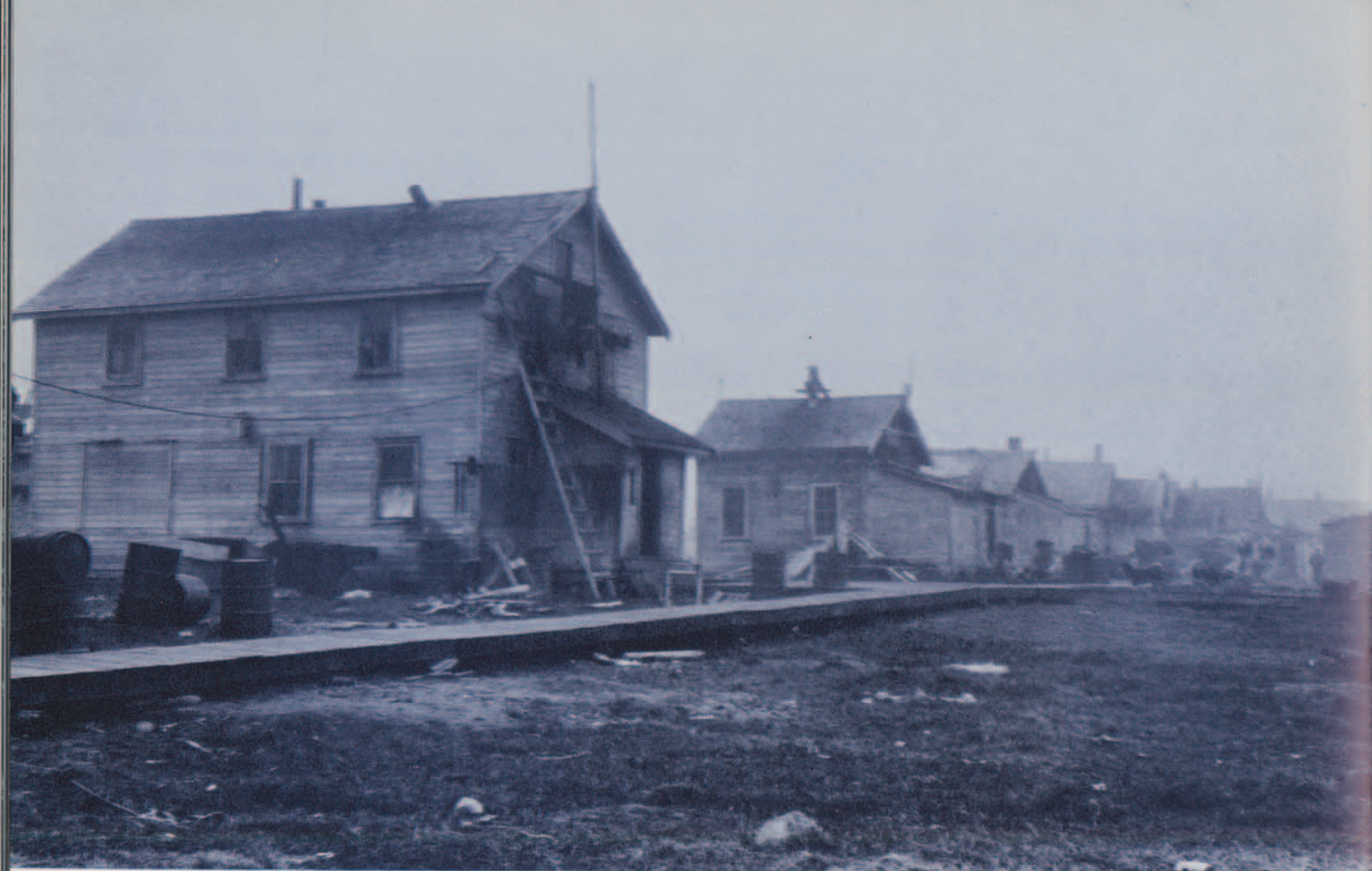
Village of Savoonga. The houses face seaward. Storm sheds protect the interior from winter winds and serve as storerooms.
