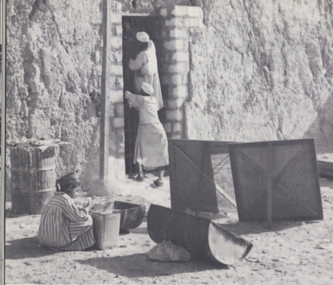
Two large reflecting mirrors stand temporarily idle while laborers attach screen across rebuilt entranceway in forecourt of tomb of the High Priest Bekenkhons (35). On their left, one of the wooden poles carrying electricity to the site. Boy is sifting, washing, and drying sand (in split barrels and metal can) to be combined with slaked lime (in standing barrel) in preparation of plaster for repairing damage to decorated walls and ceilings of subterranean chambers of the tomb.
