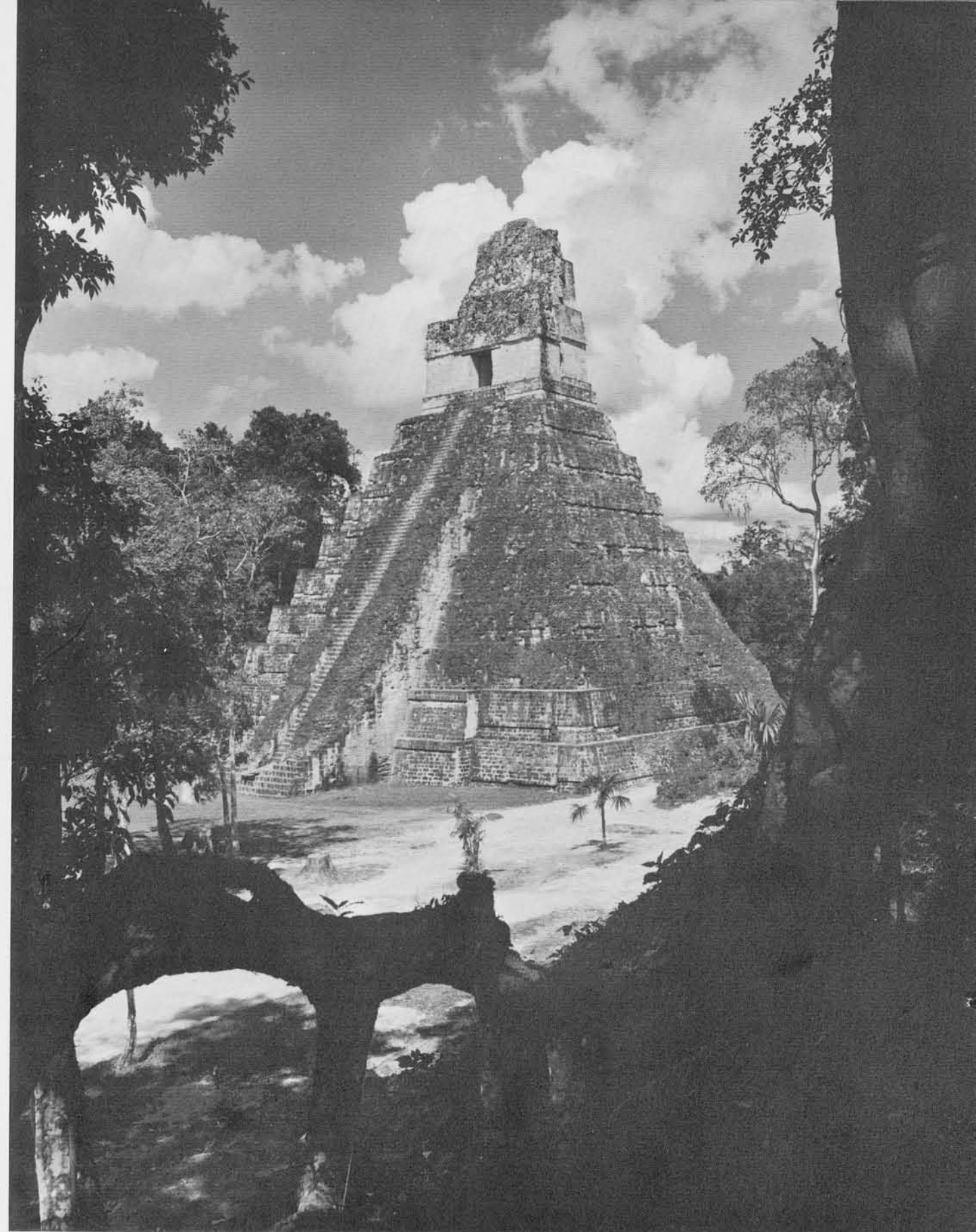
Temple I, one of the first buildings to receive attention in the program of preserving for the world the great architectural wonders of Tikal.
