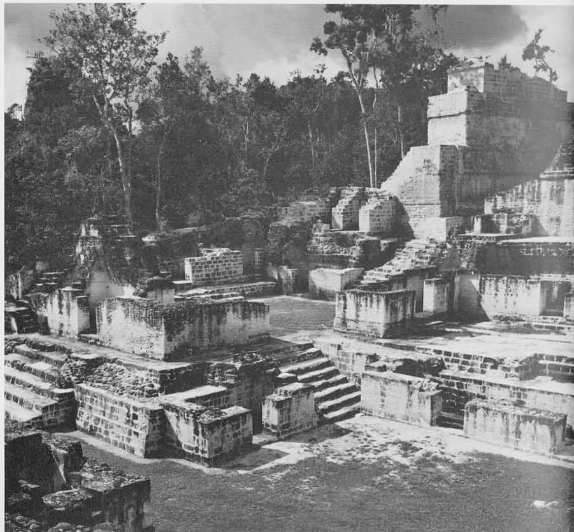
(Above right and right) Views of the recent masonry repairs conducted throughout the four and a half acres of the Central Acropolis at Tikal.
