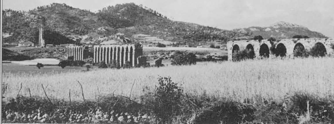
Remains of the aqueduct at Aspendos, Turkey, possibly of the third century A.D. On the low plateau to the left at the foot of the hill, beside the house, stand the remains of the north pressure tower. From a reservoir atop this hill the water flowed down and across the aqueduct bridge, then up again to another reservoir on the south pressure tower. In effect this was a siphon.
