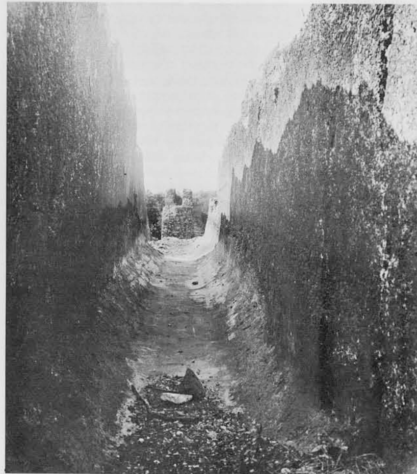
Water channel of the Minturnae aqueduct showing the cement lining.
