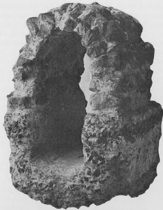
Section of the underground aqueduct at Cologne, Germany, late first century A.D. The bed and lower portion of the walls are of rubble and cement while the upper sections of the walls and the vault are of stone with cement mortar. The lower part of the channel is lined with cement.
