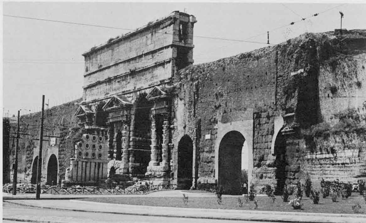
The Porta Maggiore at Rome with the stone channels of the Aqua Claudia and the Aqua Anio Novus atop the ornamental gateways.
