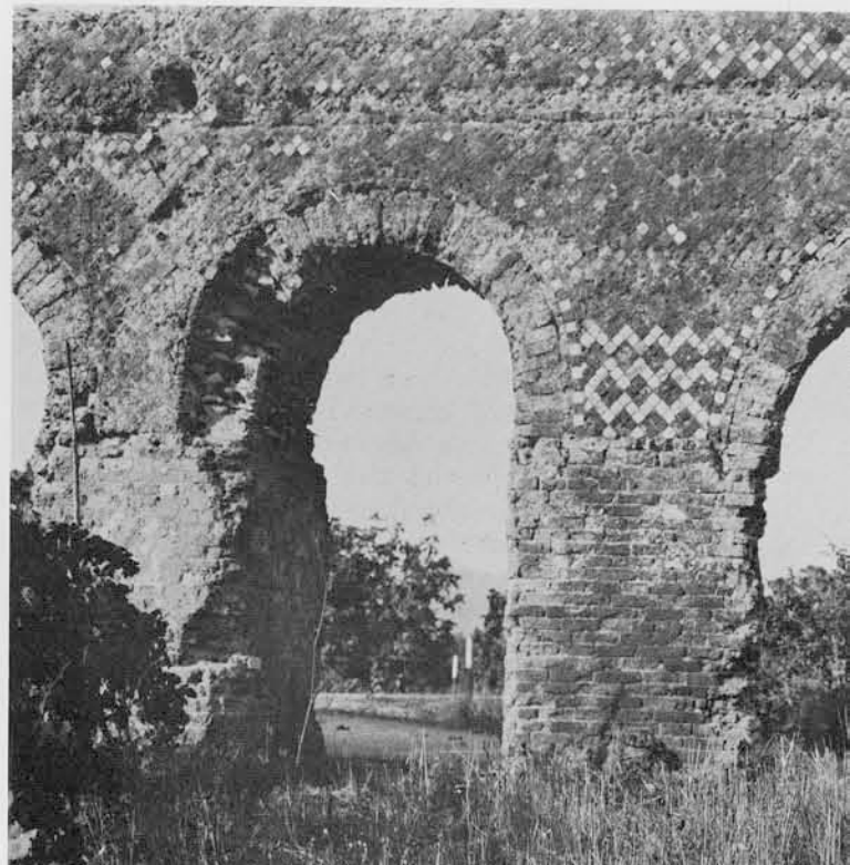
Aqueduct at Minturnae, Italy, dating to the Augustan period (27 B.C.-A.D. 14). The facing is of brick and tufa covering a rubble and cement core. The mosaic pattern in the tufa work is unusual.
