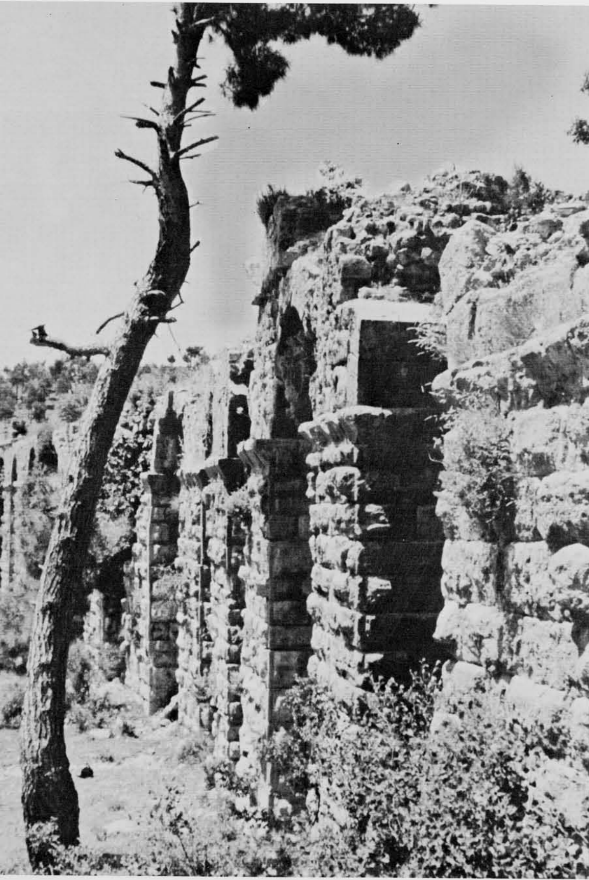
1 The Side Aqueduct. Part of the aqueduct remaining downstream from the prospective dam.
