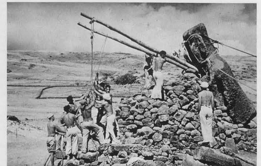
7 Twelve men, using poles, stones and ropes, raised this statue into position in 18 days. (Heyerdahl, Aku-Aku , pp. 194-95; reproduced courtesy of the Kon-Tiki Museet, Oslo, Norway)
