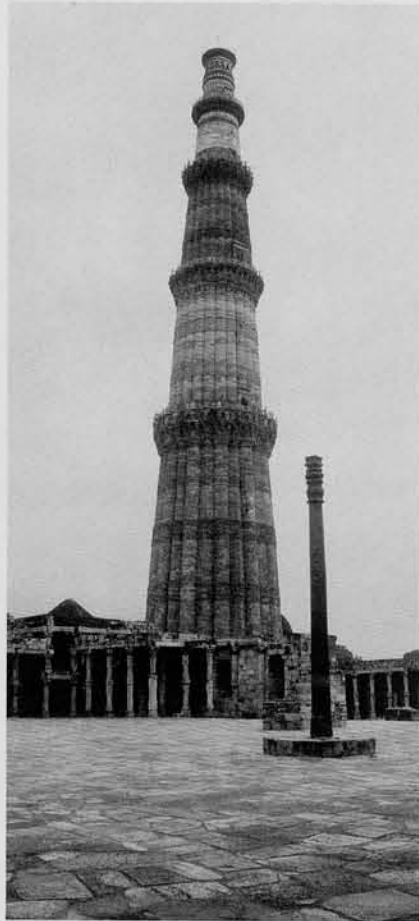
4 The Delhi pillar. A metallurgical analysis done in 1912 determined that the pillar was made of 99.72 percent pure iron, with 0.1 percent phosphorus, 0.006 percent sulphur, and traces of carbon and silica. (Photograph by Robert Raymond)
