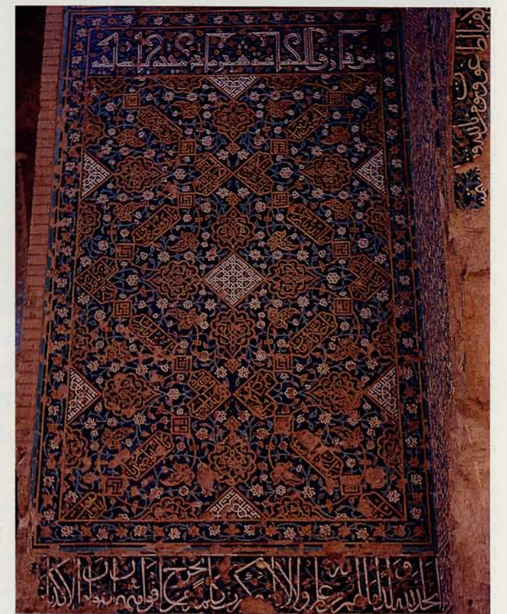
14 Mosaics made of brick, plaster, and glazed faience tiles began to be used in the decoration of major buildings in Iran during the 7th/13th century. The "Blue Mosque" (Masjid-i Janhanshah) in Tabriz, finished in 870 A.H./1465 A.D., provides some of the most beautiful examples of this kind of tilework, employing both Decorative Kufic and Tholth inscriptions. The building was destroyed by an earthquake which leveled the city in 1194 A.H./1780 A.D. (Photo courtesy of M. M. Voigt)
