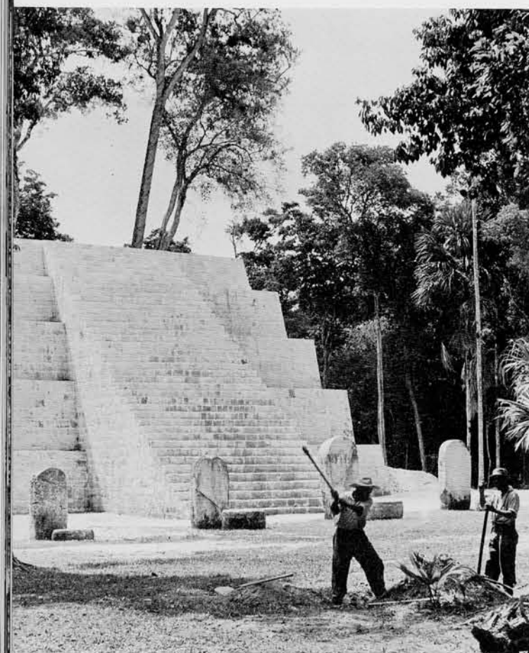
(Above) Collapse of repaired walls of Structure 78 due to torrential rains. (Below) The same area showing the final clearing of stumps and leveling before the repaired stelae and pyramid.
