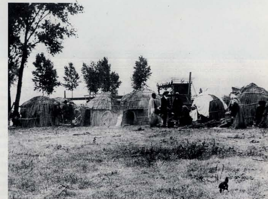
FIG. 4. TEMPORARY VILLAGE OF TULLE HOUSES constructed on the lake shore in Lakeport. Traditional Pomo houses were made of hollow tulle rushes which provided insulation against cold and heat.
