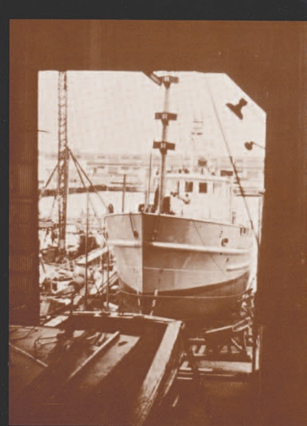
Work at the shipyard lasted into the night
