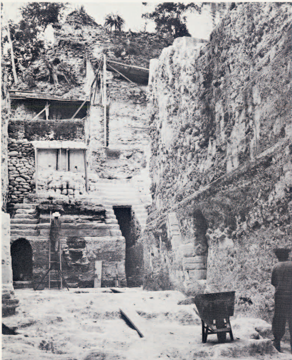
The North Acropolis trench, on completion (1963), looking north. The workman to the right is standing on bedrock while the other workman ascends ladder to Structure 5D-Sub.1-1st.
