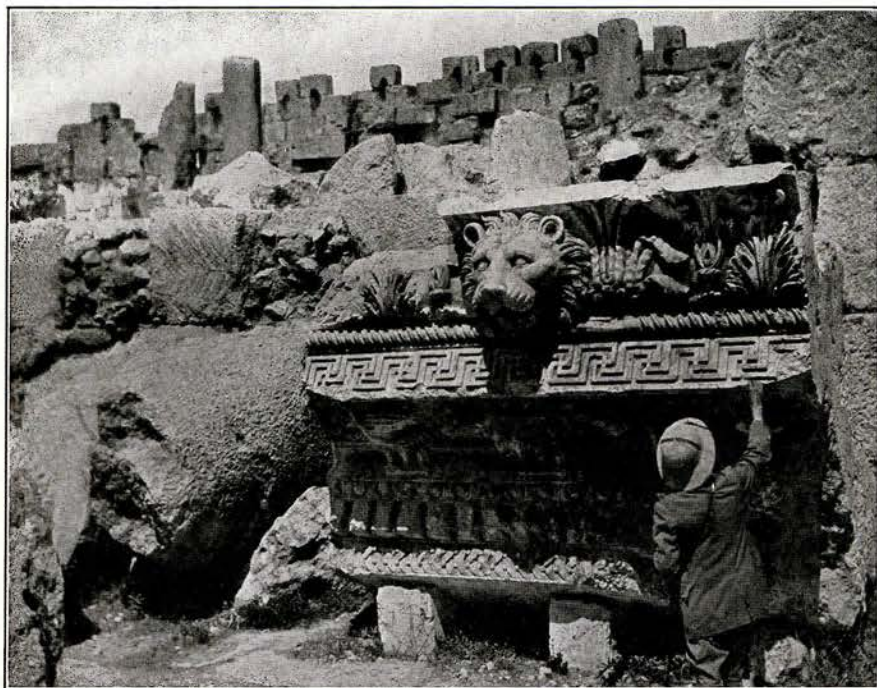
A fragment of the cornice on which lion heads placed at intervals served as gargoyles to carry off the rain water from the roof.
