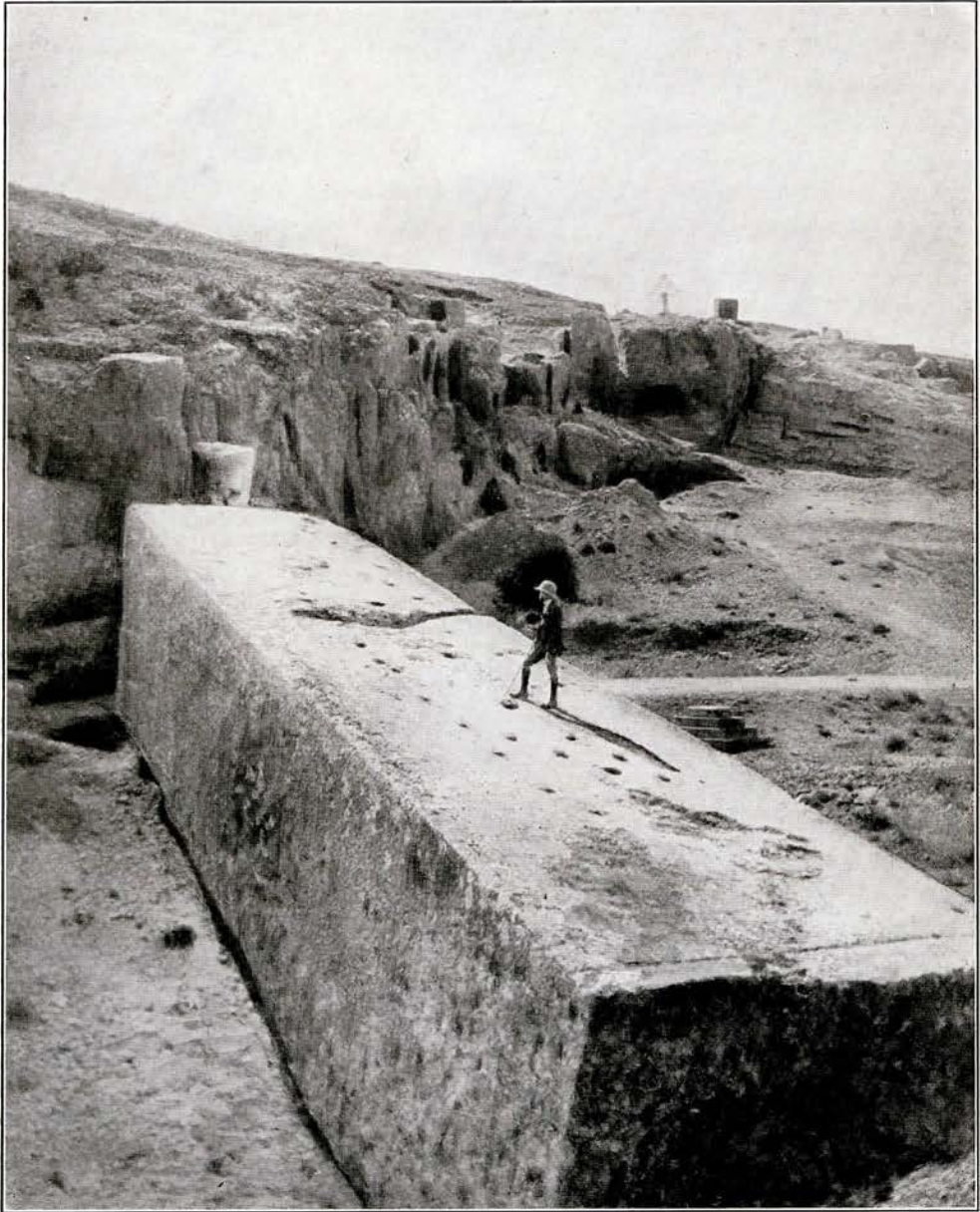
At the entrance to the quarry we find a stone 16 feet high, 16 feet wide and 69 feet long and it weighs 1500 tons. (Page 132.)
