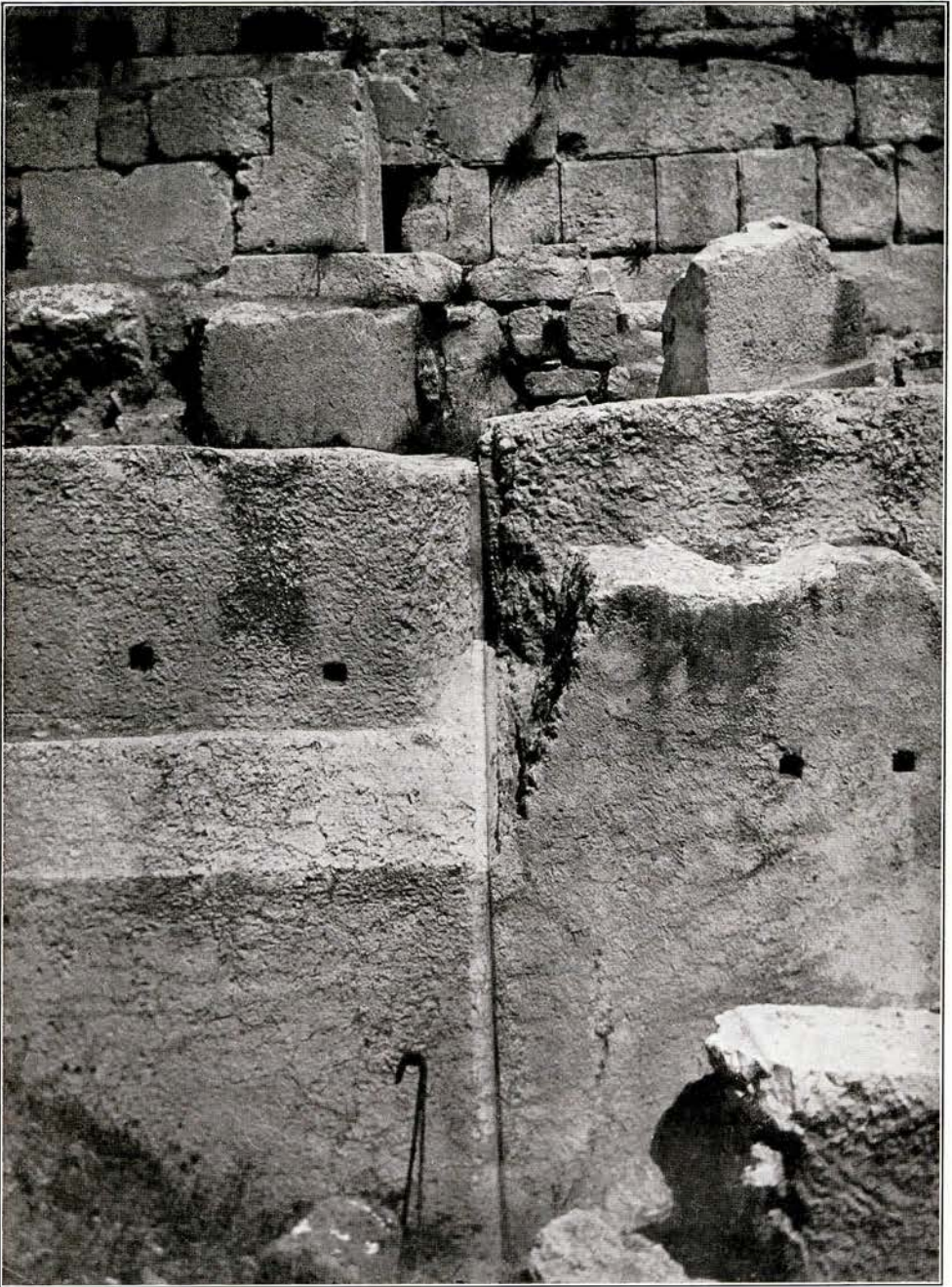
What you see is a vertical V shaped groove with polished sides at the place where the two stones come together and the joint is so fine that it is invisible to the eye. (Page 134.)
