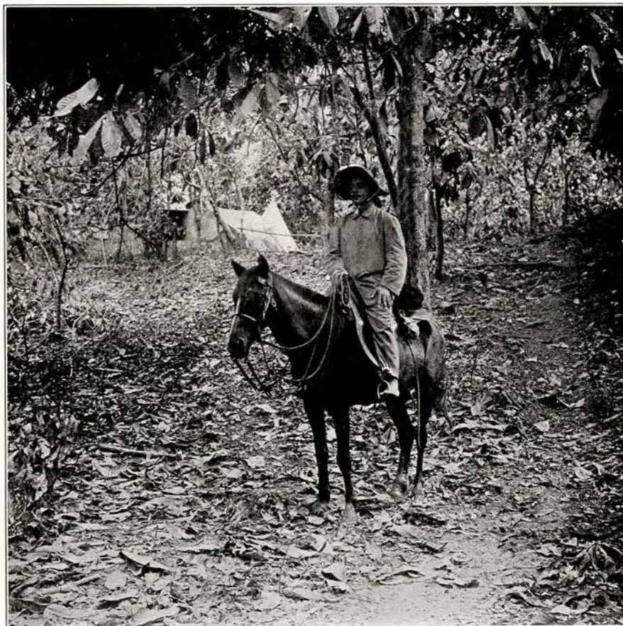
Mr. Bertino Miranda at the foot of mound excavated at Forteleza.
