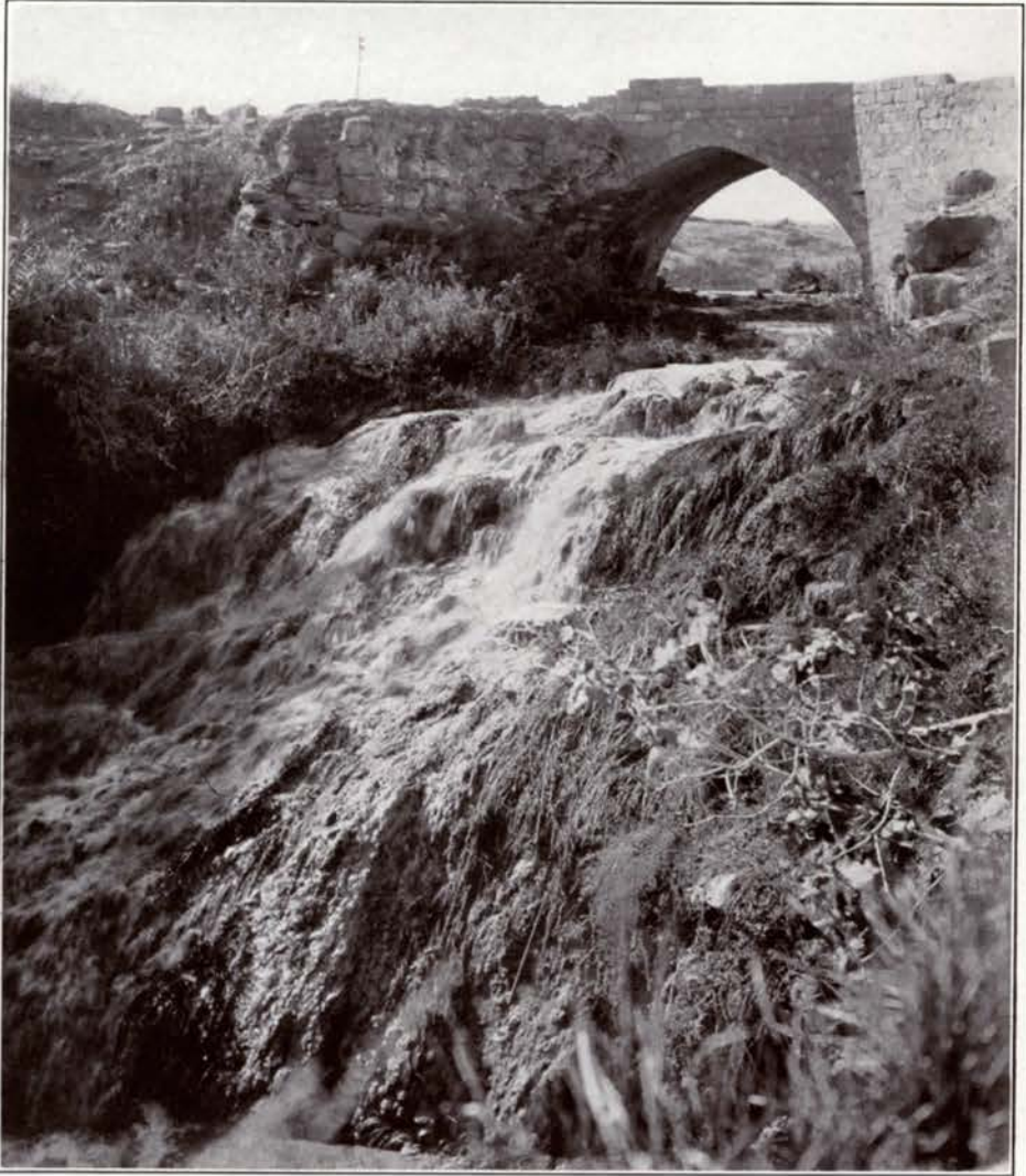
View of the Roman Bridge, with Arabic superstructure, over River Jalud, just below the Expedition House.
