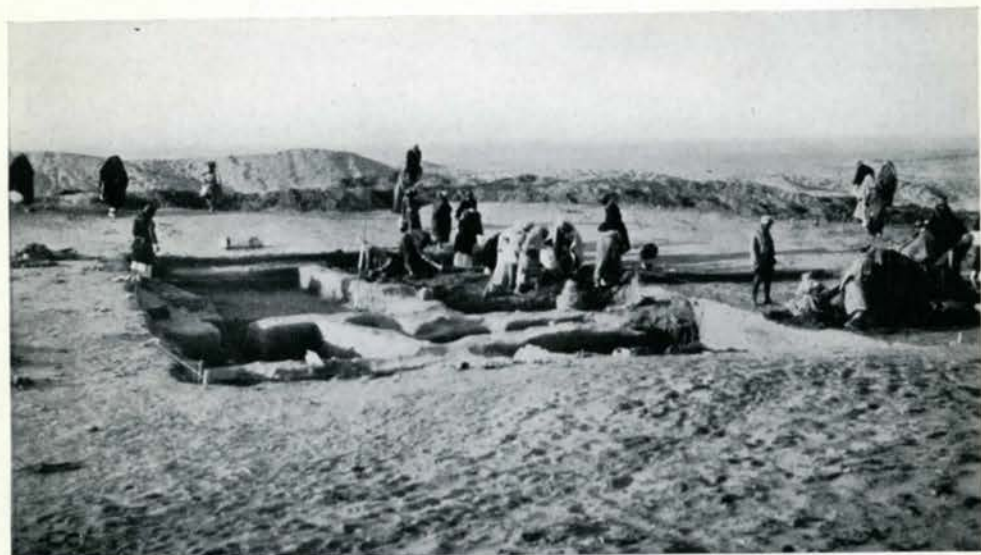
FIGURE 1.—Plots III 48, 58 excavated, HI 47 started.
