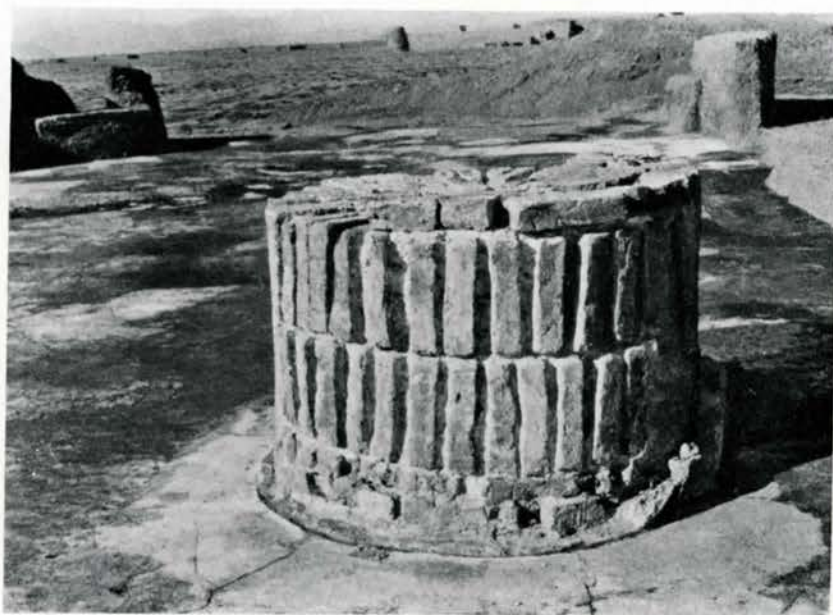
B. —SASANIAN PALACE COLUMN FRAGMENT, SHOWING TYPE OF CONSTRUCTION
